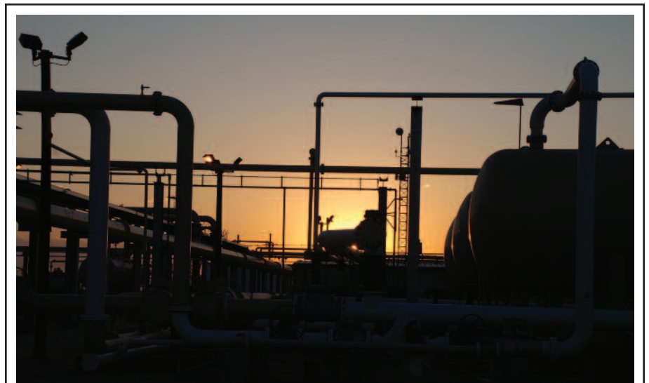
The refrigerated fractionation system utilizes a tightly integrated system of heat exchangers and separators to minimize utility costs and allow customized propane recovery levels. The first plant to use the new process was located in Sweetwater County, Wyo., followed by a plant in Ector County, Tx.
